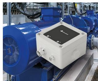
Sensor box for system monitoring
