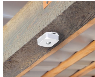
Motion detector with sensor for automatic control
