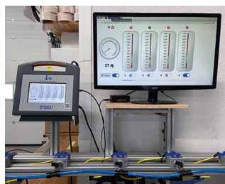
Monitoring system for cleaning nozzles
